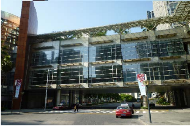
Figure 10. The arch over the municipal road
