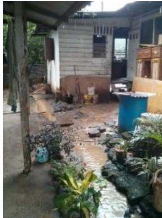
Figure 5. Infrastructure must be put into tight spaces
