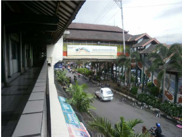
Figure 4. The feeder bridge of Beringharjo Market (source: Wisudananar, 2010)
