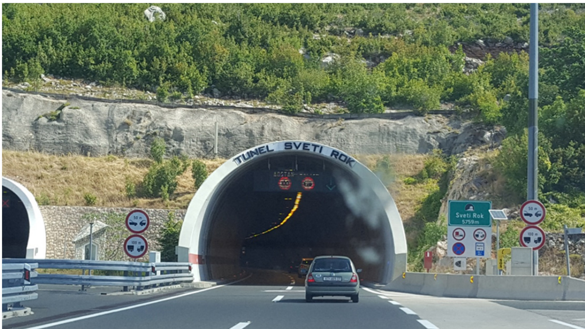
Figure 6. Road tunnel Sveti Rok
