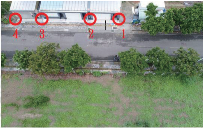
Figure 4. Feature points of the building in the experimental area
