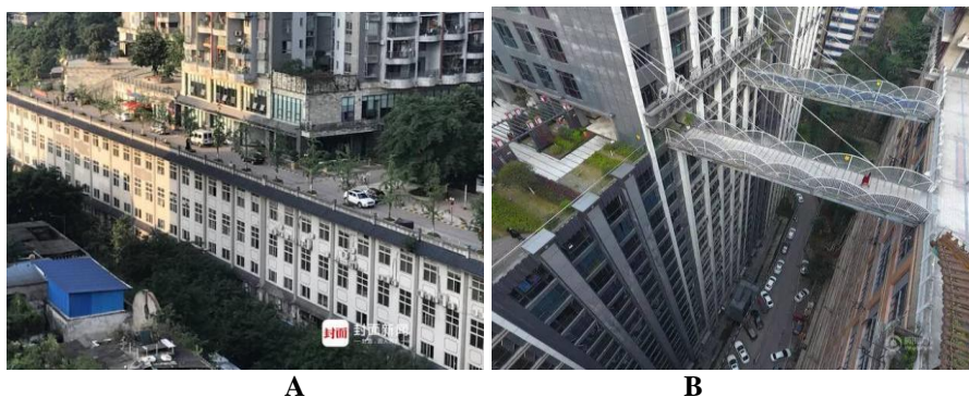
Figure 2. Different ground levels for different buildings: A) top level to ground level; B) ground level to the top level and middle level.
