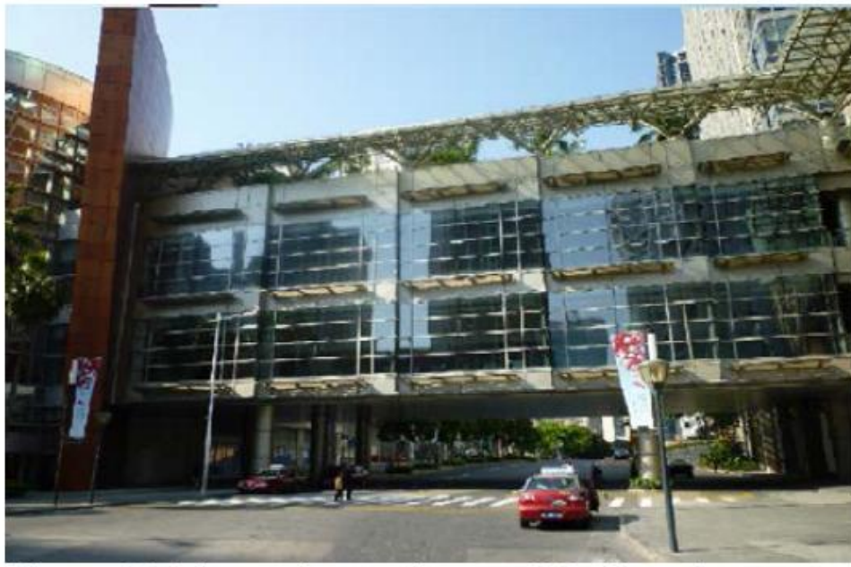
Fig. An Arch over the Municipal Road
