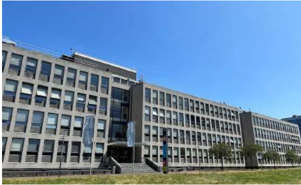
(a) the TNW main entrance
